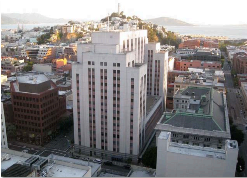
Figure 7: Photo of the exterior of the Appraisers building 4
