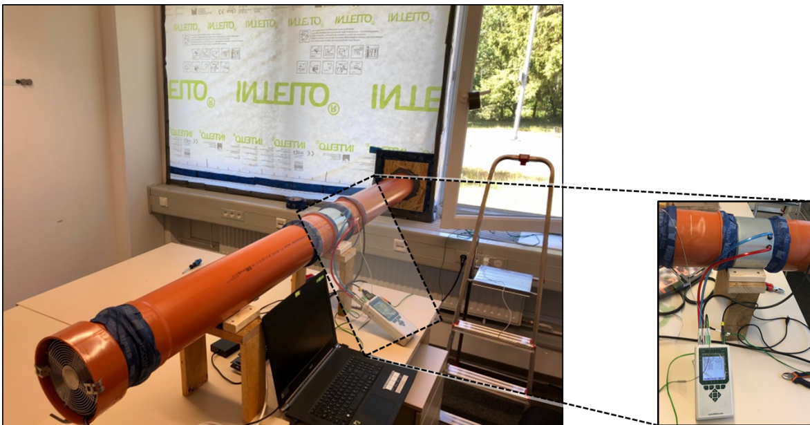
Figure 13: Experimental setup for airflow and pressure difference measurements in an office building (left) with venturi airflow meter (right)
