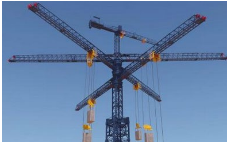
Figure 3-7. SCHEMATIC DIAGRAM OF A TOWER SGES SYSTEM AND PHOTO OF ENERGY VAULT'S SGES
