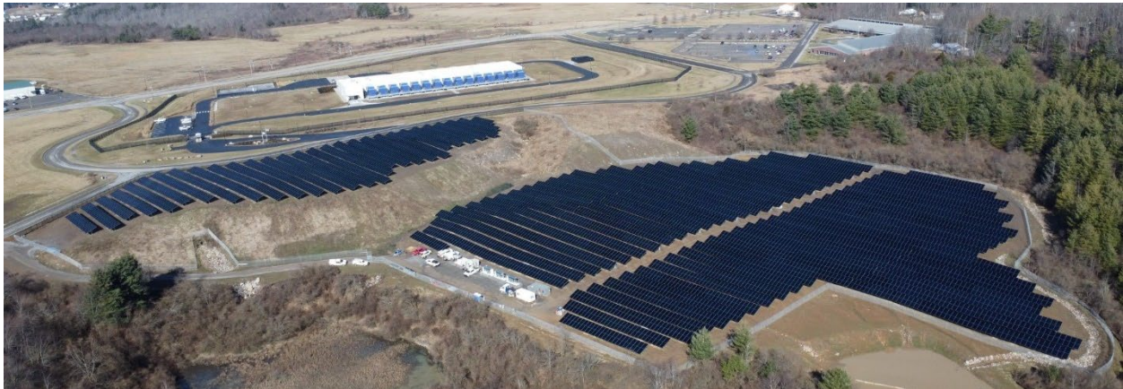
Figure 4-9. SOLAR POWERED DP MINERAL GAP DATA CENTER
