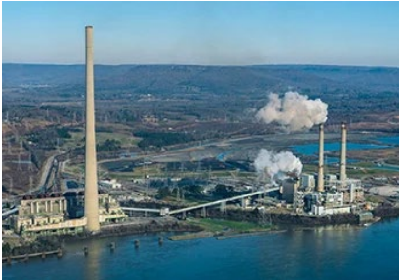
Figure 4-10. TVA'S WIDOWS CREEK COAL POWER PLANT
