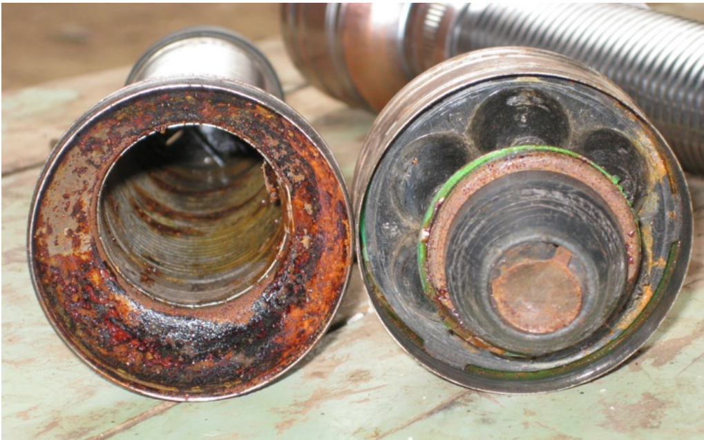
Photo 4. Corrosion from water and battery leakage.
