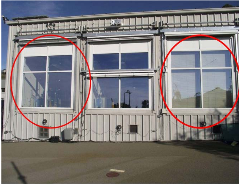
Figure 10 The Advanced Windows Test Facility at the Lawrence Berkeley National Laboratory
