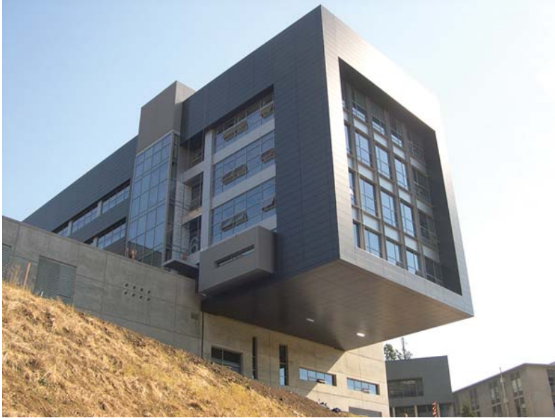
Figure 3. The Molecular Foundry at Lawrence Berkeley National Laboratory is one of many projects that have applied Labs21 EPC (precursor to the LEED-AGL) to improve the sustainability of laboratory systems.
