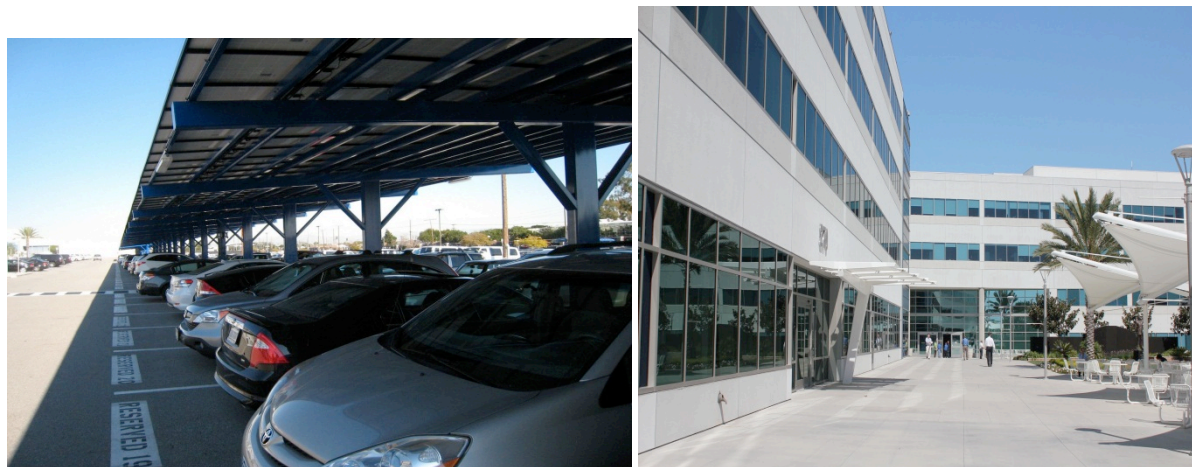
Figure 2. L.A. AFB PV canopy left and base central plaza right
