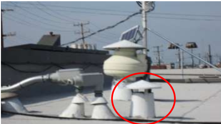
Figure 16: We located FH6's range hood outlet (circled) on its roof, but for safety reasons did not try to measure its flow
