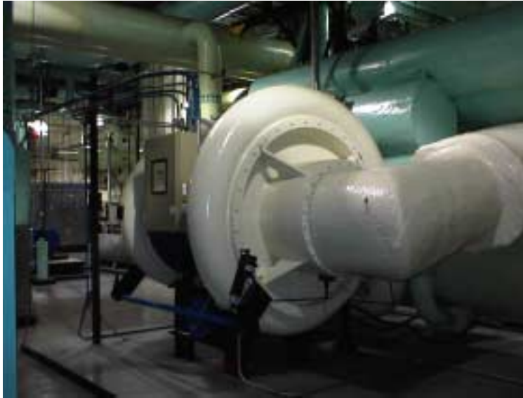
Figure 13 Centrifugal Chiller
