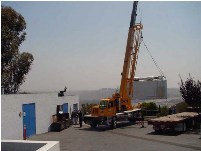
Figure 25: Placement of the Container
