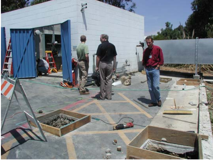
Figure 24: Generator Site During Construction
