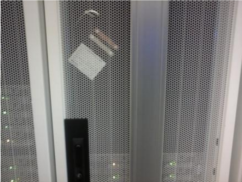
Figure 8 - Typical Coupon Mounting, Example Shown is Just Prior to Cooling Air Entering IT Equipment
