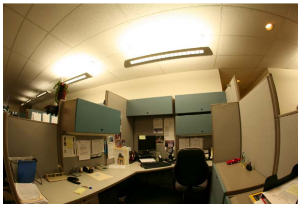
Figure 2: Cubicles lit with workstation-specific luminaires during a pilot study at the Philip Burton Federal Building.
