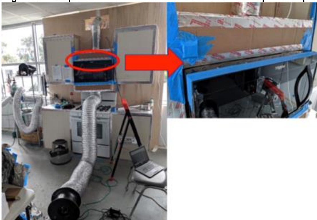
Figure 5. Example of Airflow Measurement at Inside with Top Inlet Taped
