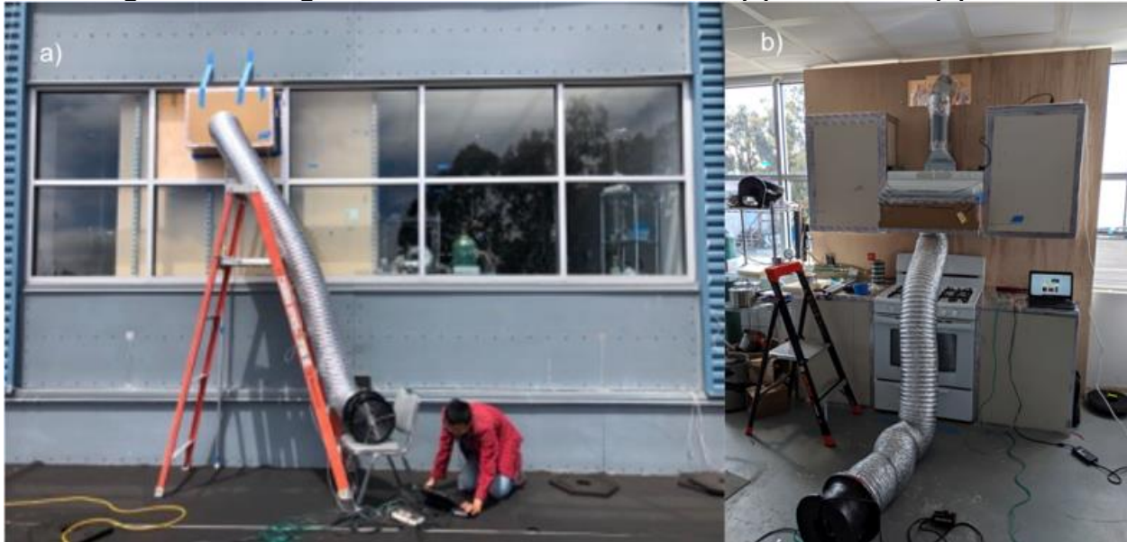
Figure 3. Configurations to Measure Airflow at (a) Outlet and (b) Inlet
