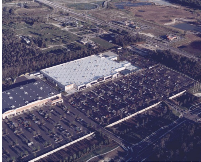
Figure 9. White roof application at large Wal-Mart retail outlet in northern California Source: Walmart
