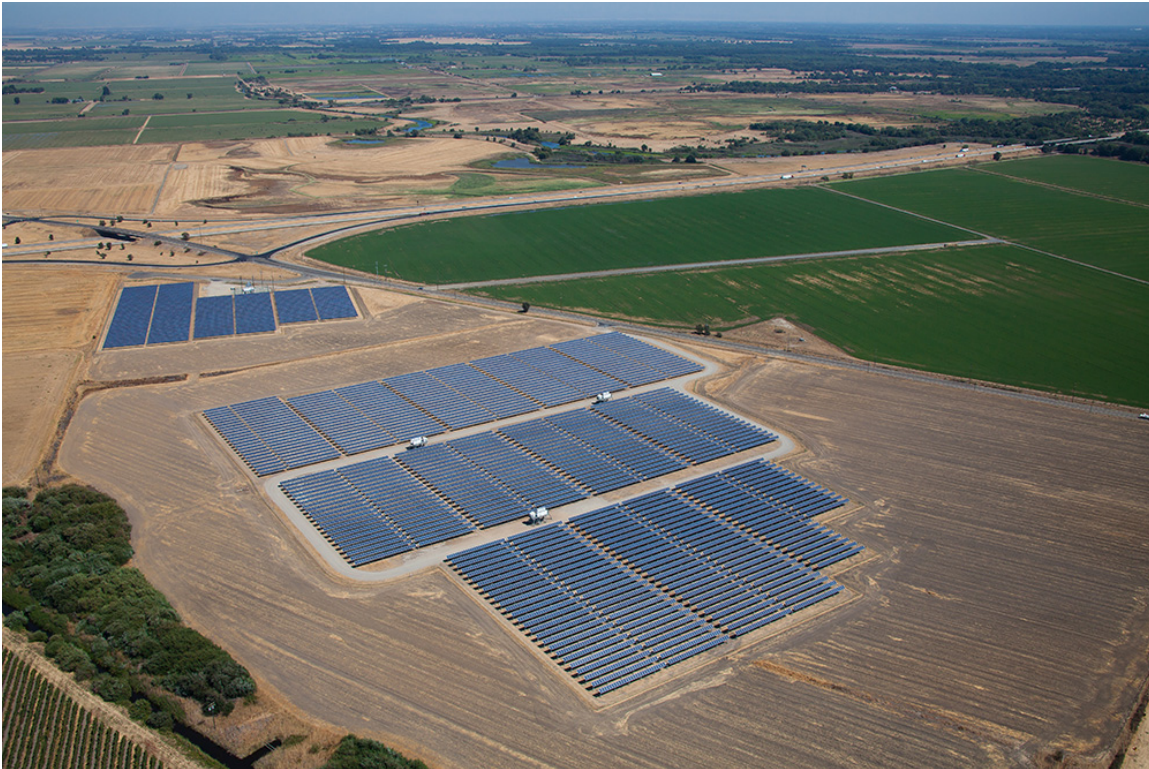
Figure 21. The 5MWp Green Acres solar PV project in Elk Grove, California
