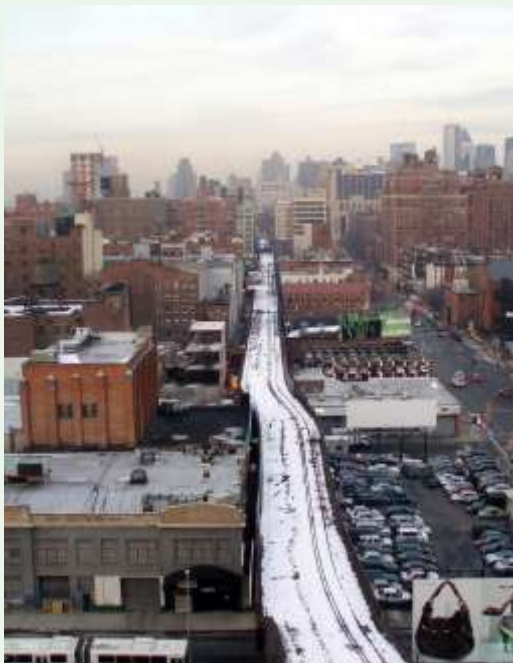
Figure 16. Before the High Line: unused elevated railway, 18th Street looking north
