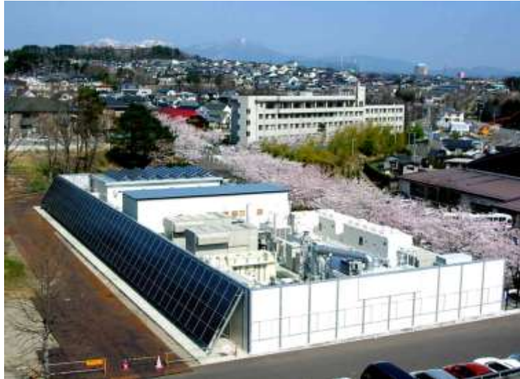
Figure 18: Overhead view of the Sendai energy center
