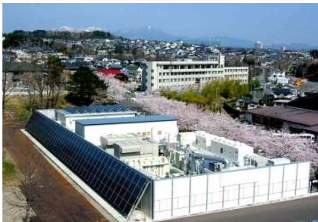
Figure 4: Overhead view of the Sendai energy center
