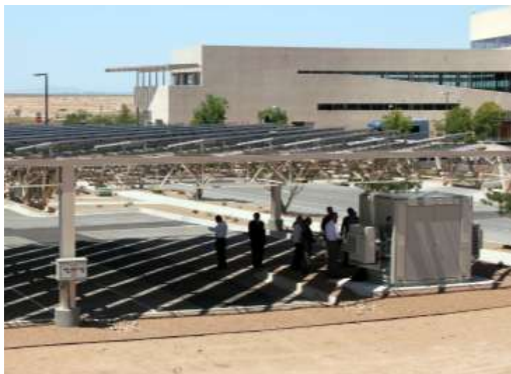
Figure 34: Solar PV array at the Aperture Center microgrid
