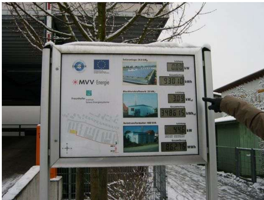
Figure 32: Energy demand and supply display at MVV microgrid project
