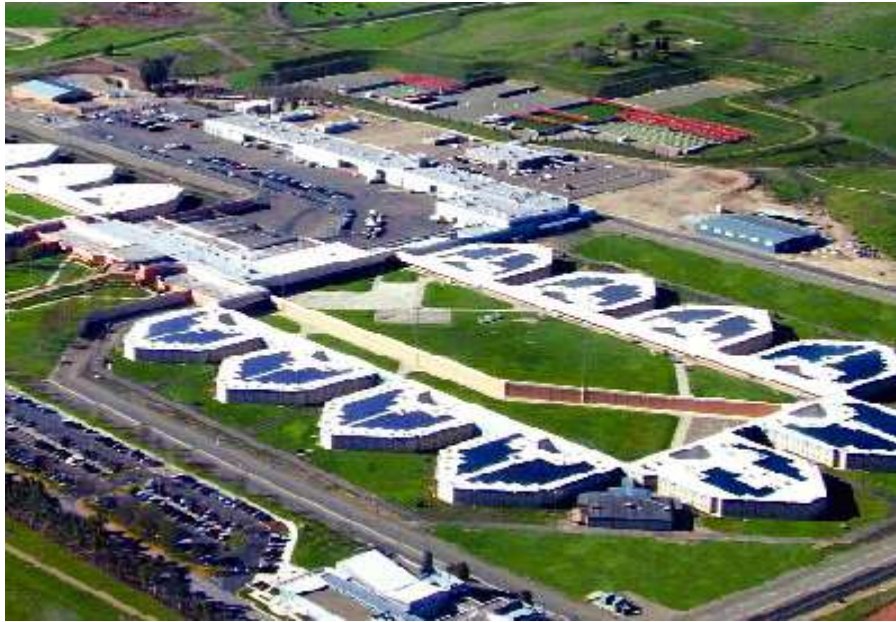
Figure 16: Overhead view of the Santa Rita Jail showing the rooftop PV array
