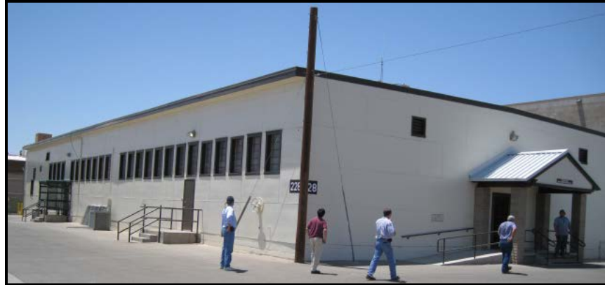
Figure-11: Building 228 at Site III (MCAS Yuma).
