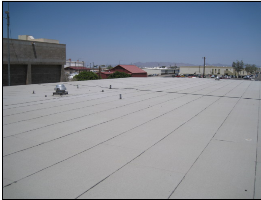
Figure-13: Rooftop photo of Building 228 at Site III (MCAS Yuma) prior to BIPV installation.
