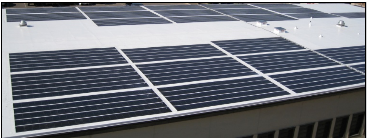
Figure-14: Rooftop photo of Building 228 at Site III (MCAS Yuma) after BIPV installation.
