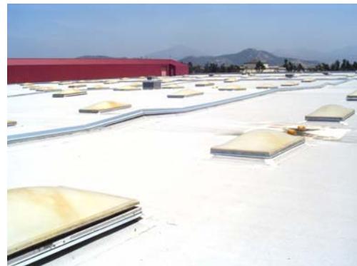
Figure 11. rooftop at the San Diego P&DC
