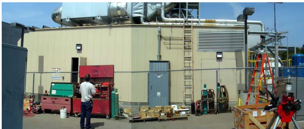
Figure 7. generator housing at the San Diego P&DC
