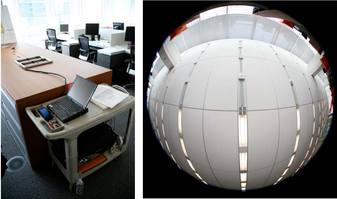
Figure 1-4. Lighting commissioning cart (left) consisting of a 3x3 array of illuminance sensors placed on the work plane to monitor average illuminance over a 20 minute period. Ceiling pattern of dimmed fixtures (right) with window at the top of the photograph.
