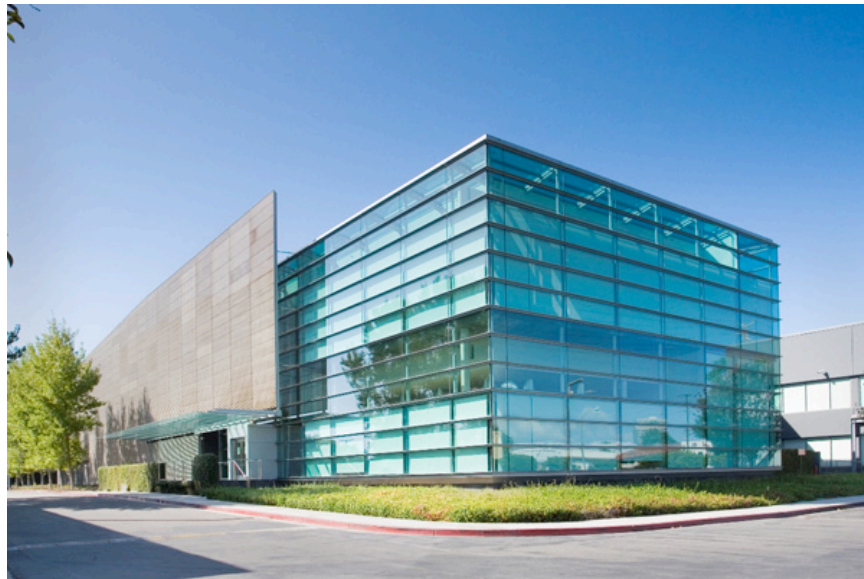
Figure 2-1: Street View of the Digital Realty Data Center, Located in El Segundo, California
