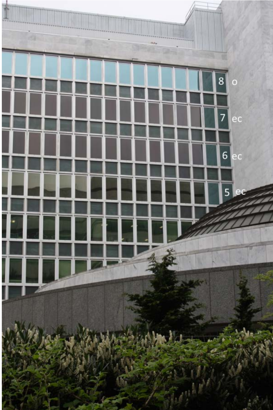
Figure 3. Photograph of the west wing of the south façade, April 9. The EC windows on Floors 6–7 were set to Tint 4 ( T_{vis}=0.02 ). The EC windows on Floor 5 were operating in the automatic mode (Tints 1–3). Floors 3–4 (EC windows not yet installed) and Floor 8 show the appearance of the original (“o”) existing reference low-e windows.
