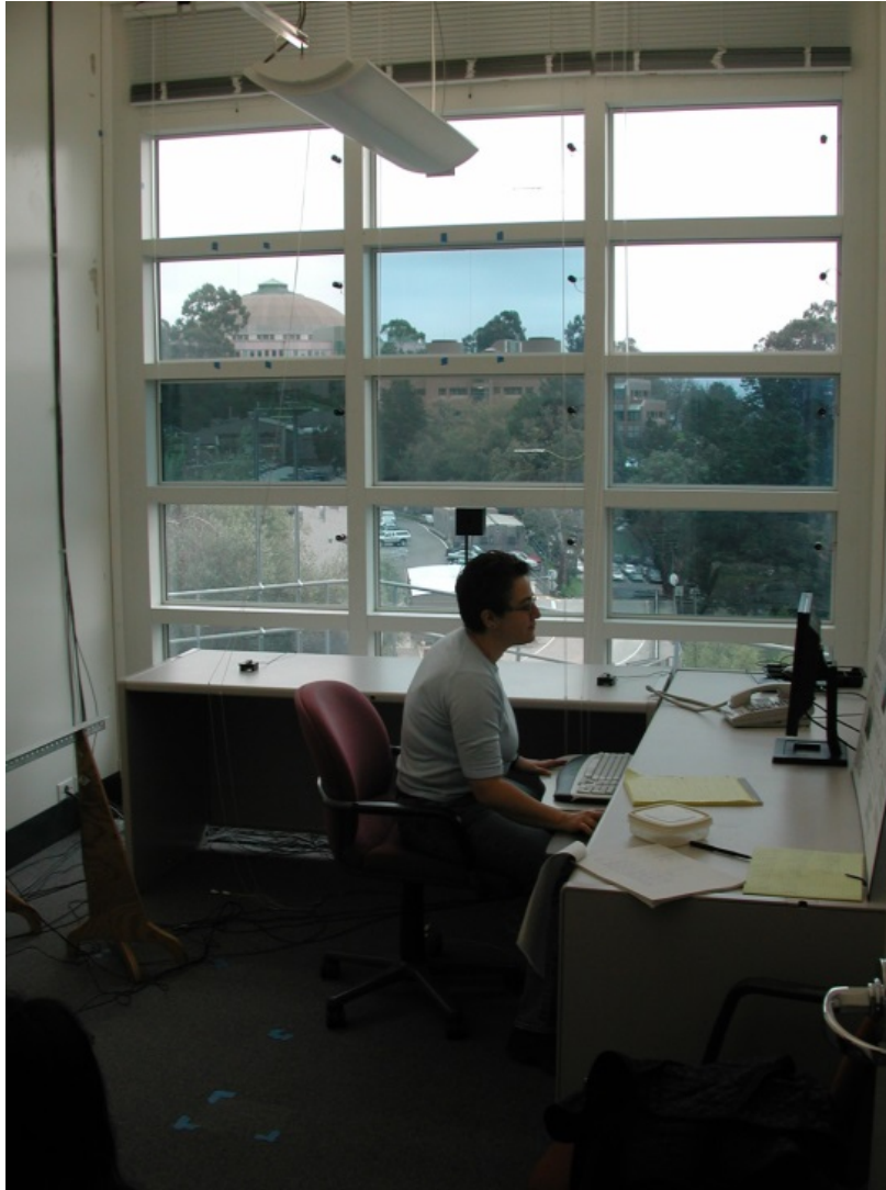
Figure 2. Occupants switched individual EC window panes to suit their preferences for view, glare control, and privacy. Image from [56].
