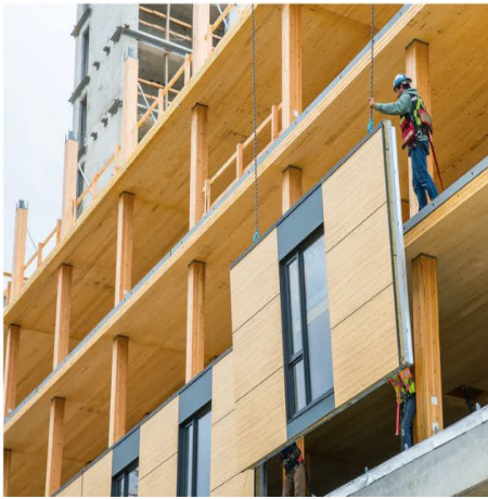
Figure 4-18. Off-site manufactured façade install
