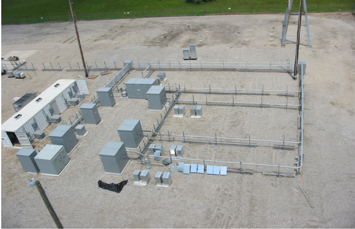
Figure 1 - CERTS Microgrid Aerial Photo
