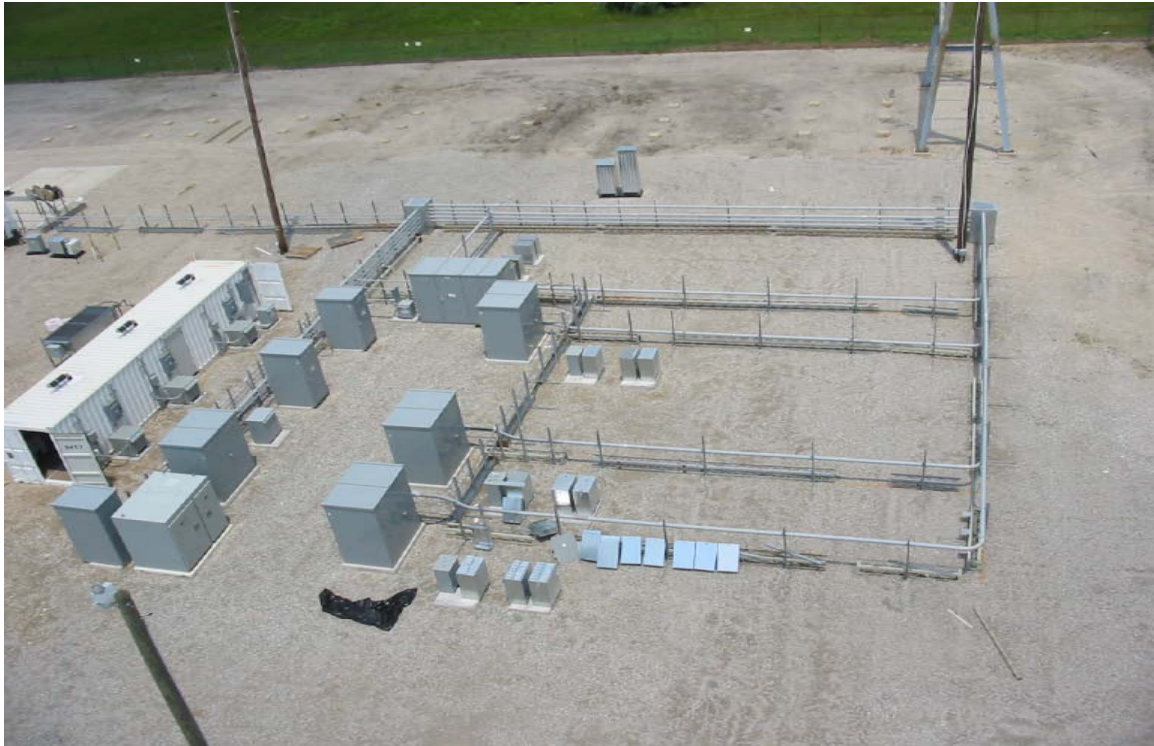
Figure 1 - CERTS Microgrid Aerial Photo
