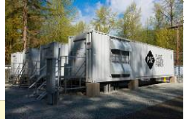
2 MW / 4.4 MWh lithium-ion/phosphate battery – Glacier, WA
