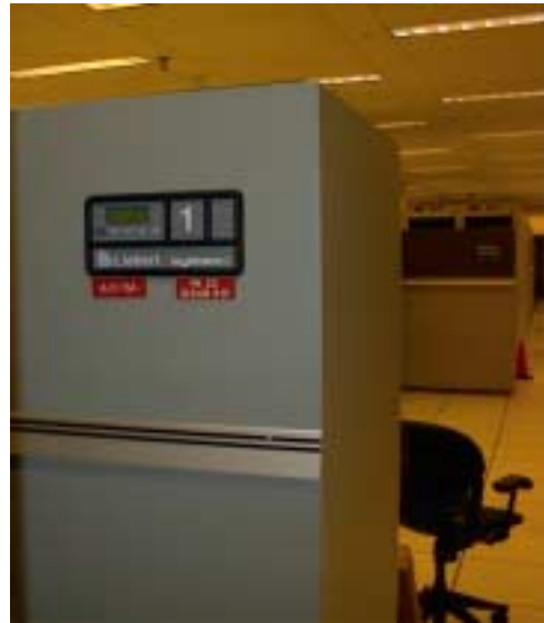
Figure 1 CRAC Unit
