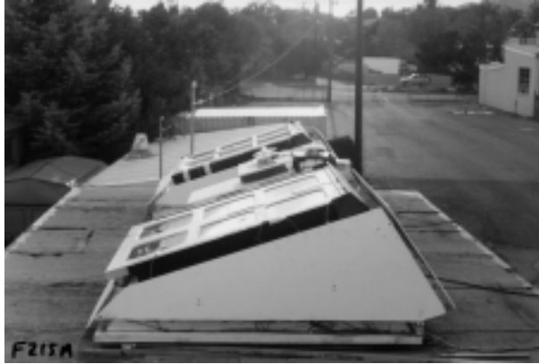
Figure 1. Skylights Mounted on Test Chambers. Electrochromic sample EC-2 is the near skylight, and the clear double glazed comparison sample is the far one. Due to the sizes of the EC-2 samples supplied, the skylight assemblage overlapped the frame by a few inches. The frame is sealed to the inner side of the glazing to cut off this extra area (not visible in the photograph). White sun shields shade the exterior of each skylight well adapter. Between the two skylights are a pyranometer measuring total horizontal solar irradiance, and two instruments tilted to measure total irradiance on the sample plane. One of these is a pyranometer; the other is a solar-blind pyrgeometer measuring long-wave infrared radiation. The latter is the nearer of the two instruments and has a dark dome.
