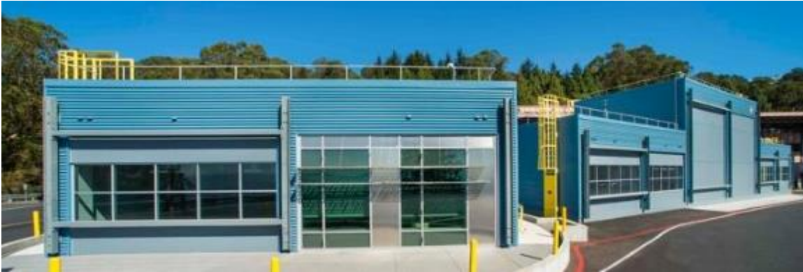
FIGURE 1. GENERAL VIEW OF THE CLIMATE TEST ROOM
