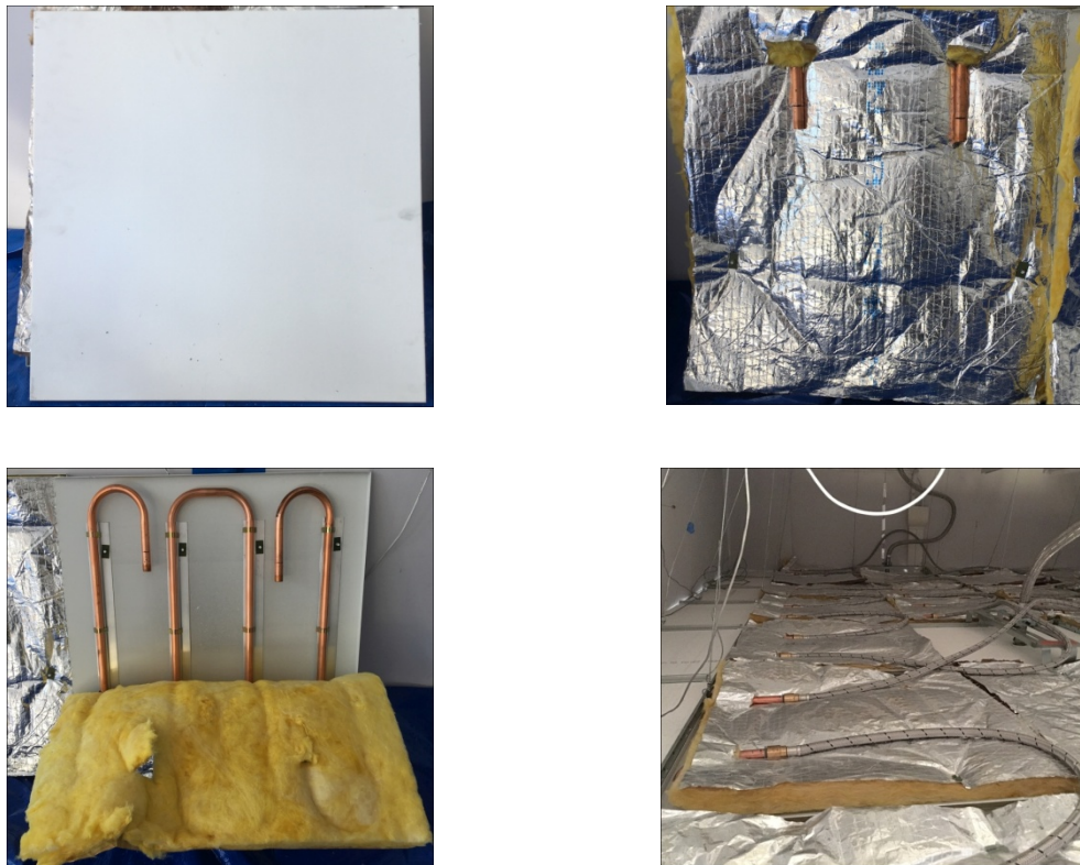
FIGURE 3. RADIANT CEILING PANELS: FRONT (UPPER LEFT), BACK (UPPER RIGHT), PIPING (LOWER LEFT), CONNECTIONS (LOWER RIGHT)
