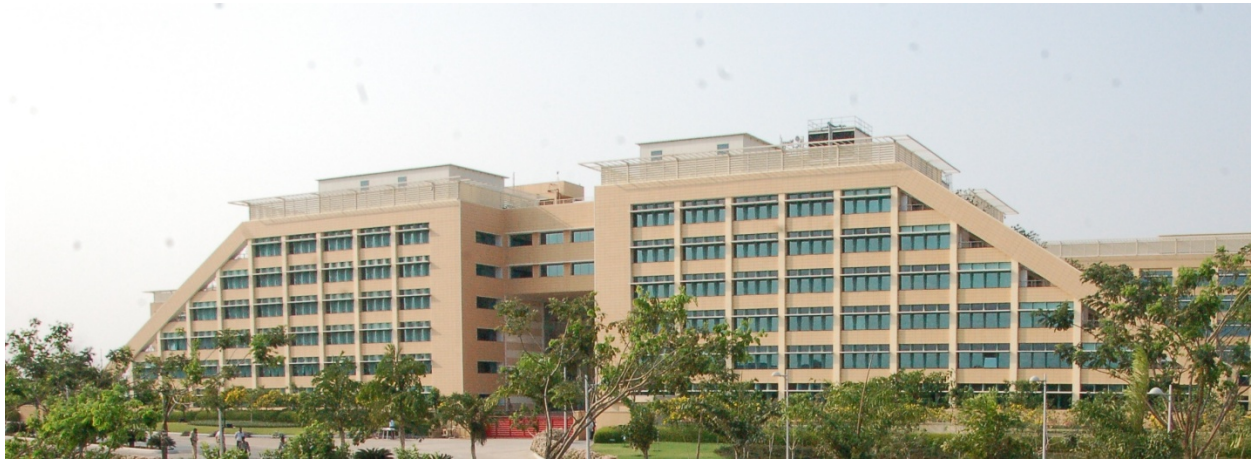
FIGURE 322 THE OFFICE BUILDING IN HYDERABAD, INDIA USED TO COMPARE THE ENERGY PERFORMANCE OF A RADIANT SLAB TO A VAV SYSTEM
