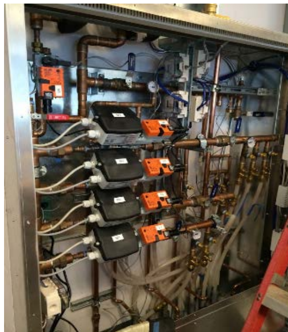
FIGURE 6. THE RADIANT SYSTEM CONTROL PLUMBING
