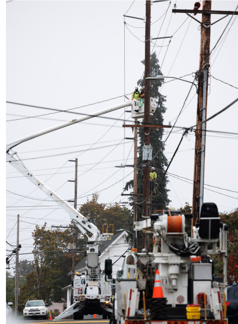
Line Crew Construction – Portland General Electric
