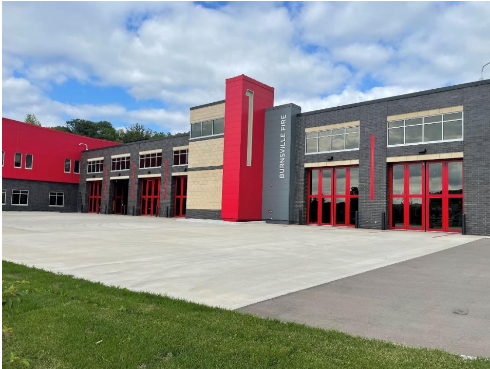
Fire station 1 at 14275 Newton Ave, Burnsville
