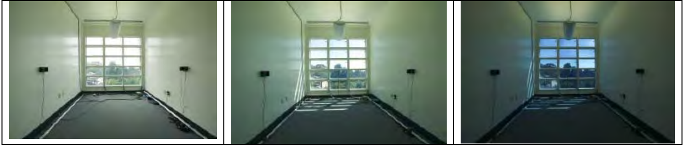
Figure 3 New LBNL facility for comparative field tests of advanced facades. Electrochromic glazings are controlled real-time to meet design illuminance but control solar gain and glare. Left: Under cloudy conditions the glass is at maximum transmittance. Center: When sun comes out the window begins to darken. Right: After 5 minutes the window is fully darkened but the lights are on to meet illuminance levels.
