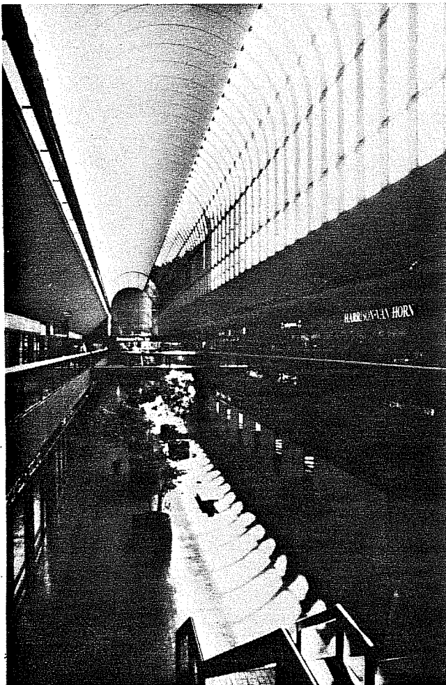
A continuous clerestory above the two-story central space of the Pacific Design Center in Los Angeles lends dramatic emphasis to the geometry of the space. Direct sunlight in this instance enhances the visual drama without being a detriment to activity. Diffuse light from this central area spills into adjacent showrooms.
