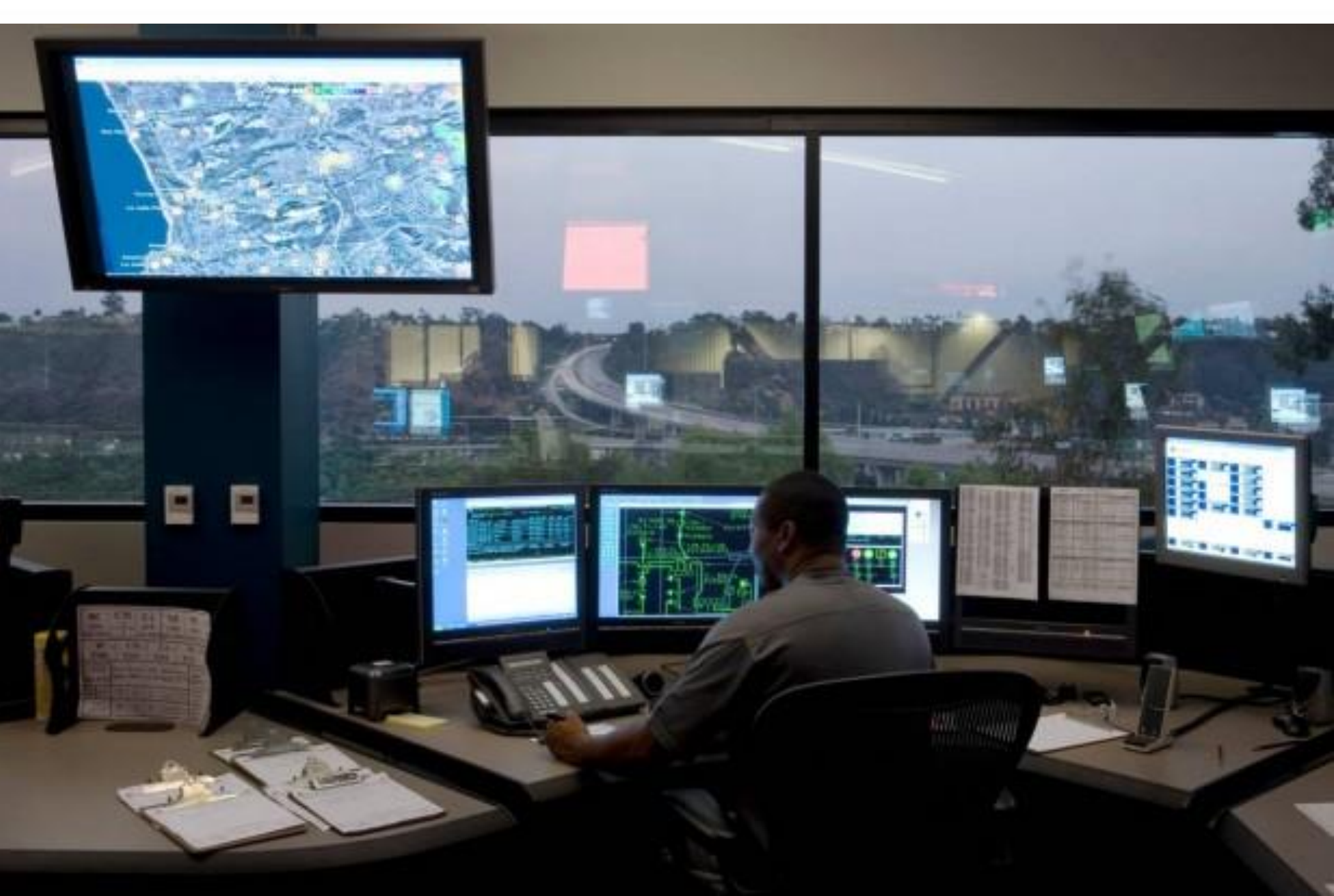
newer DO control room at SDG&E
